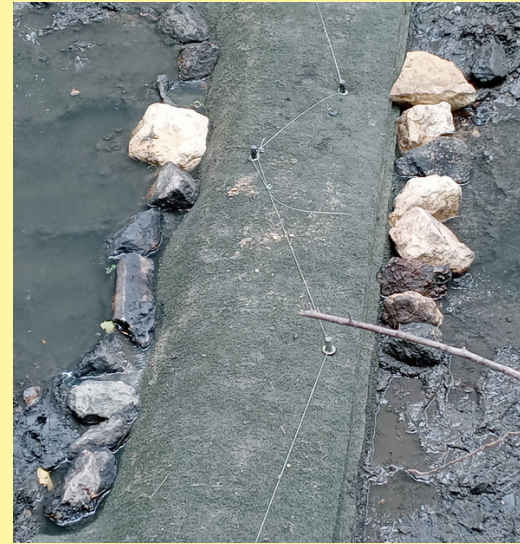
Biofilter Installation
